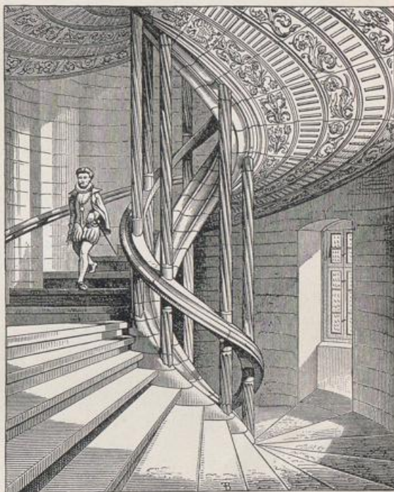
Abb. 159. Treppe in Mergentheim.
