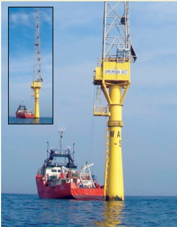
Abb. 1: Messmast Amrumbank West.
