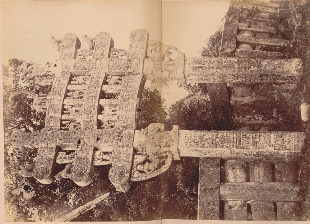
FRONT VIEW OF NORTHERN GATEWAY.
