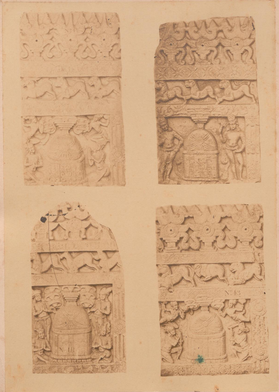
PORTIONS OF FRIEZE OF CENTRAL BUILDING.
