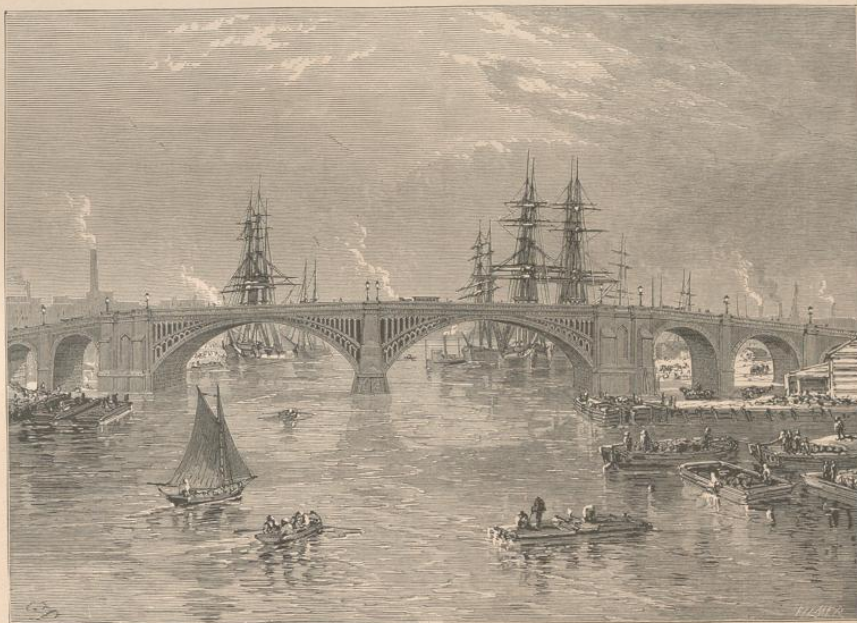
Chestnut-Street Bridge, on the Schuylkill.
