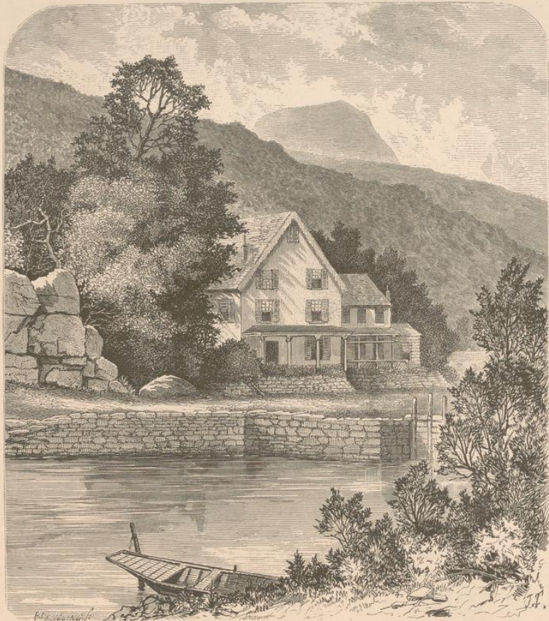
Terrace House and Thorn Mountain.
