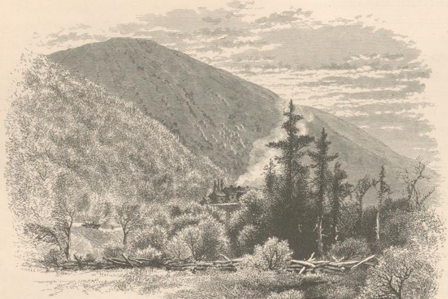
Hoosac Mountain and Tunnel Works.
