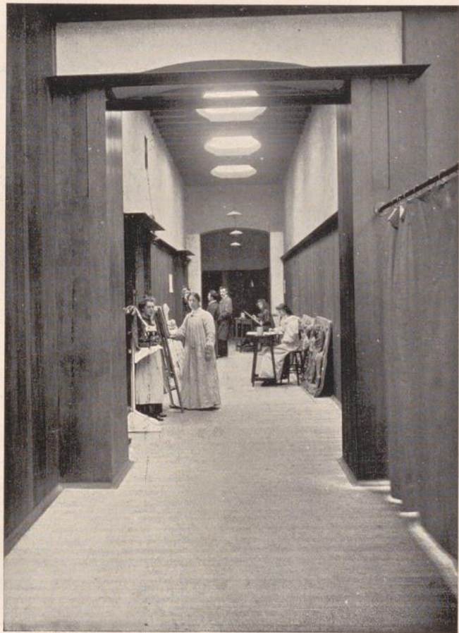
GLASGOW SCHOOL OF ART; FIRST FLOOR CORRIDOR
