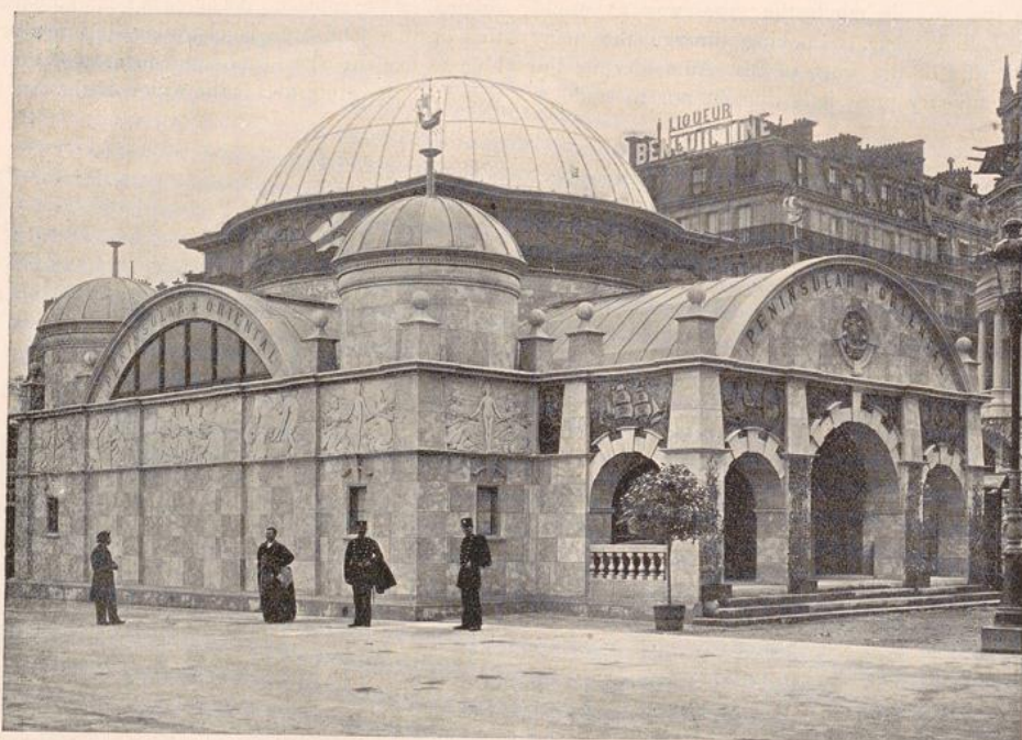
PENINSULAR AND ORIENTAL PAVILION (ENTRANCE FRONT)
