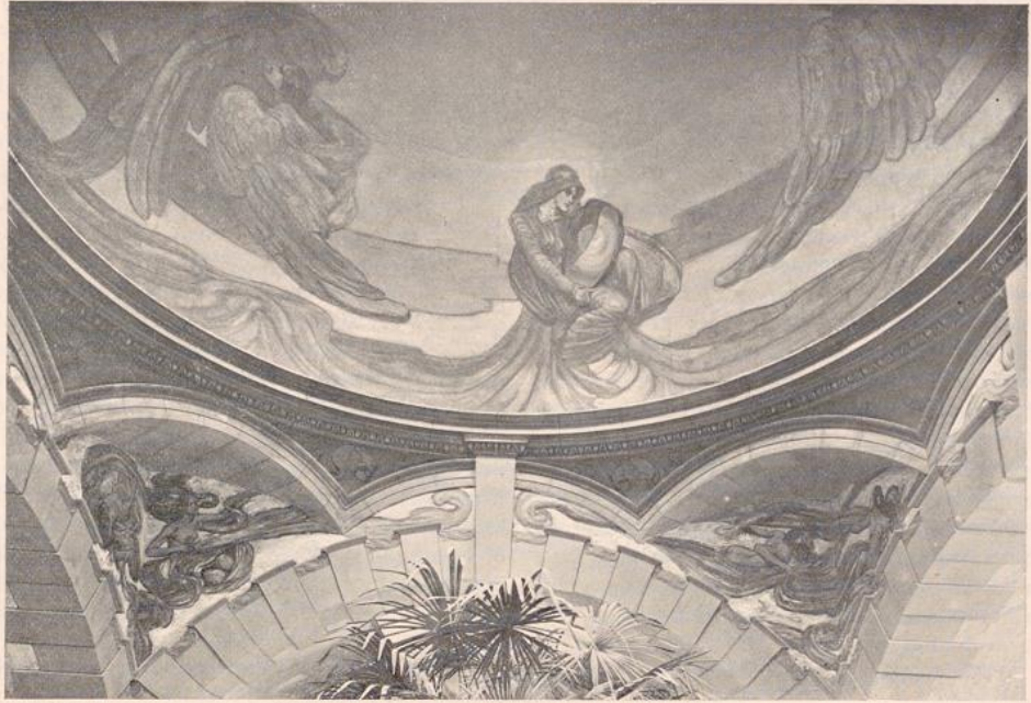
PORTION OF DOME, SHOWING POSITION OF SPANDRELS
