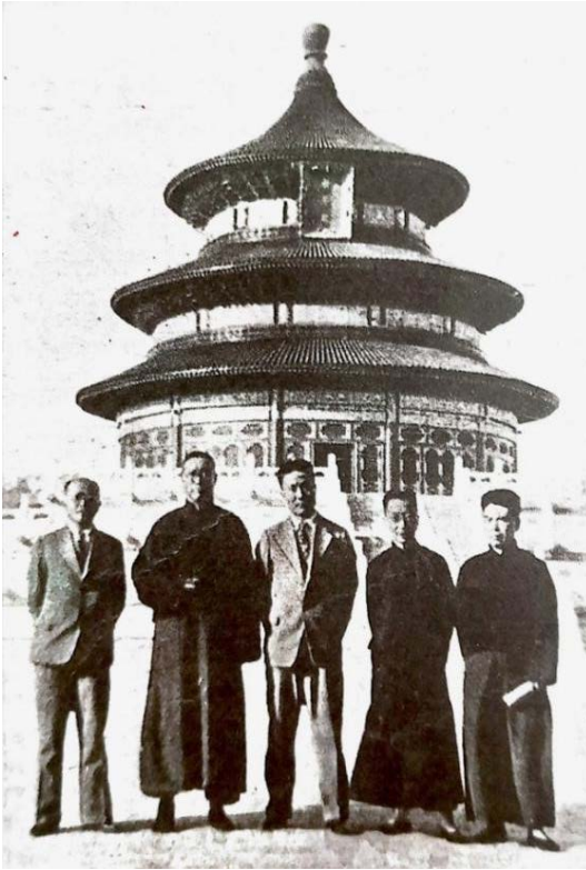
Abb. 7: As a member of the standing committee, Teng Ku on behalf of the central government inspected the renovation of cultural heritages such as the Temple of Heaven and the Forbidden City in Beijing, October 1936. (Teng Ku is standing in the middle)
