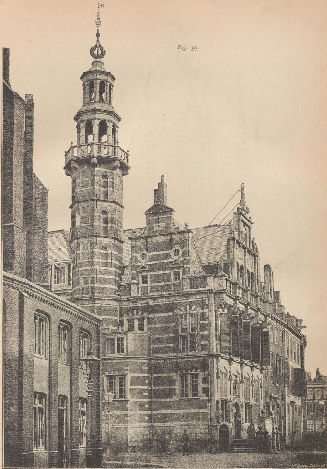
Rathhaus in Haag 90 ).
