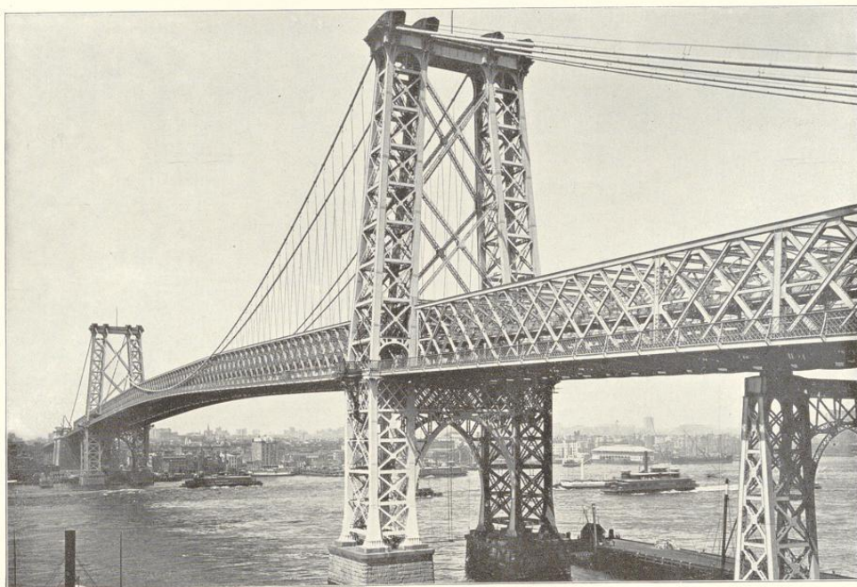
Abb. 91. Williamsburg-Brücke in New - York. 1896—1903. By Detroit Photographig Co.
