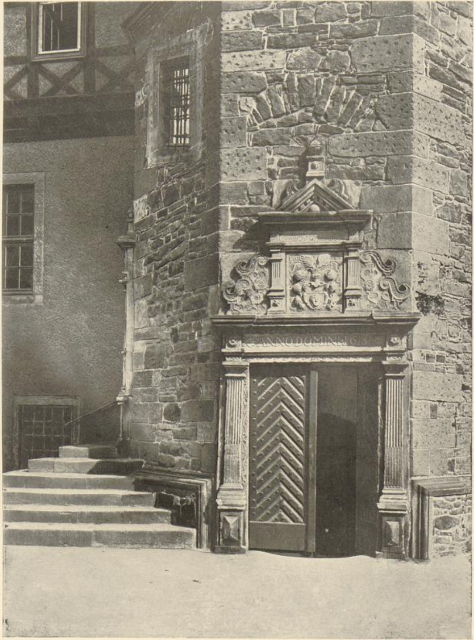
16. Rathaus in Höxter. Tür am Treppenturm.
