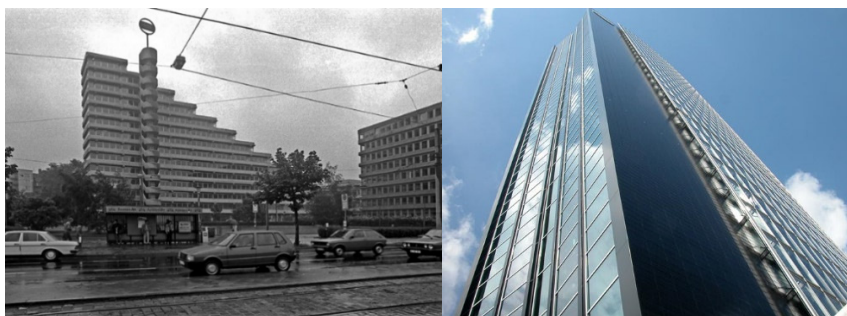
Figure 11: ARAG Buildings from 1966 and 1999
